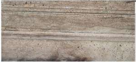
SINCE THE CONSTRUCTION OF THE PALACE WAS WAY BACK IN OLD TIME THE TIMBER HAS BEEN DETERIORATED BY THE PEST ATTACK . SEVERAL SPOTS OF PEST INVASION IS OBSERVED ALL THROUGH THE TIMBER FRAMES.
