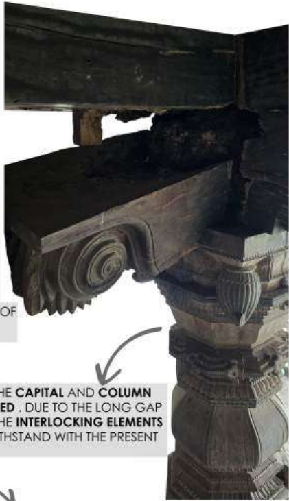
SINCE THE CONSTRUCTION OF THE PALACE WAS WAY BACK IN OLD TIME THE TIMBER HAS BEEN DETERIORATED BY THE PEST ATTACK . SEVERAL SPOTS OF PEST INVASION IS OBSERVED ALL THROUGH THE TIMBER FRAMES.
