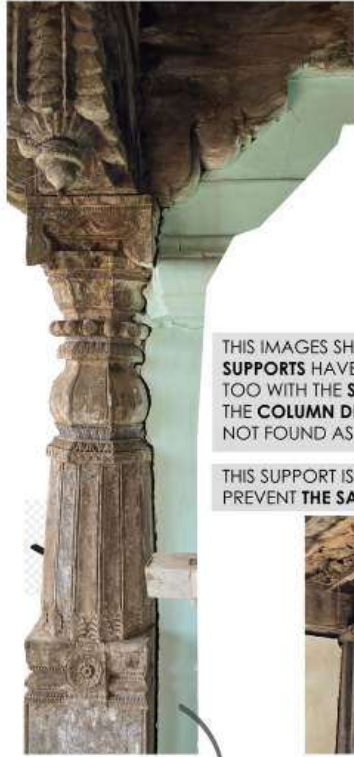
THIS IMAGES SHOWS US HOW THE COLUMN MADE OF TIMBER AND THE WALL MADE UP OF MUD - HAS BEEN DETACHED OVER THE TIME. THIS IS BECAUSE OF WEATHERING AND NO MAINTAINANCE CARRIED OUT .
