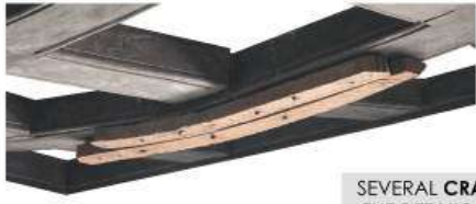
THESE PICTURES TELL ABOUT THE SAGGING IN THE CEILING WHICH ARE REINFORCED BY THE EXTERNAL SUPPORTS .
