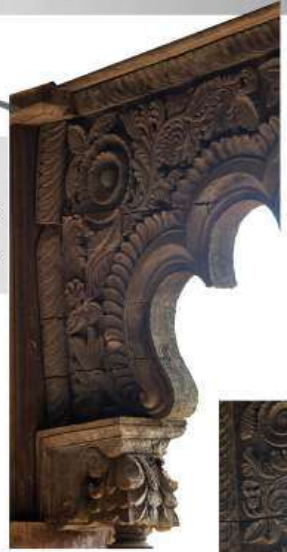
SEVERAL CRACKS ARE BEING OBSERVED ON THE DETAILS OF THE ARCHES OF THE FRONT FACADE . THIS IS BECAUSE OVER THE TIME, MAINTENANCE HAS NOT BEEN CARRIED OUT AND THE TIMBER IS EXPOSED TO VARIOUS HARSH CLIMATIC CONDITIONS , LEADING TO THE CRACKS AND BREAKAGES .
