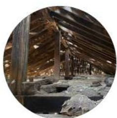
SPACE BETWEEN ROOF AND ATTIC
