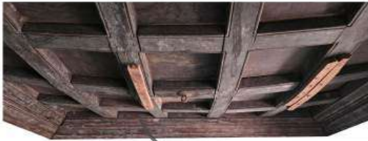
THESE PICTURES TELL ABOUT THE SAGGING IN THE CEILING WHICH ARE REINFORCED BY THE EXTERNAL SUPPORTS .
