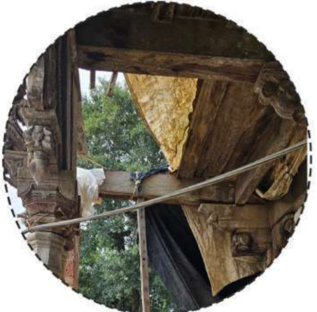
DAMAGED ROOF STRUCTURE
