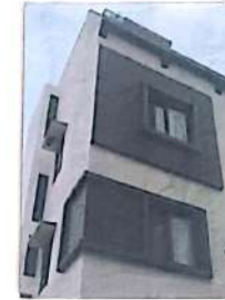
VIEW OF FUNDERMAX CLADDING
